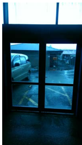
Fire Exit to West
