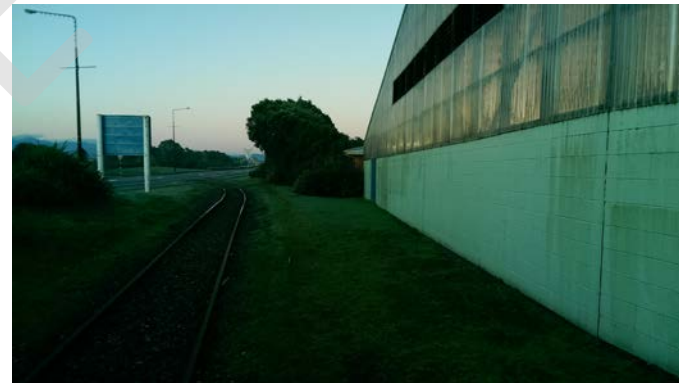
Eastern Façade and Railway Line
