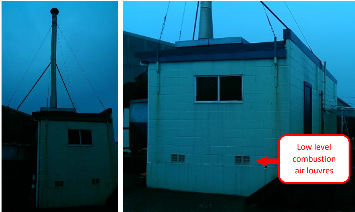
Picture 3: Boiler Plant Room
