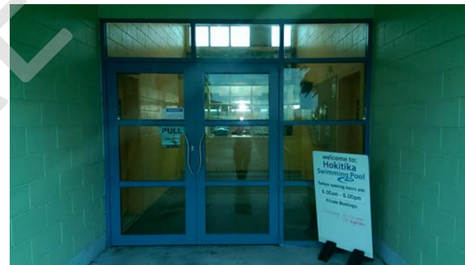
Main Entry Pools
