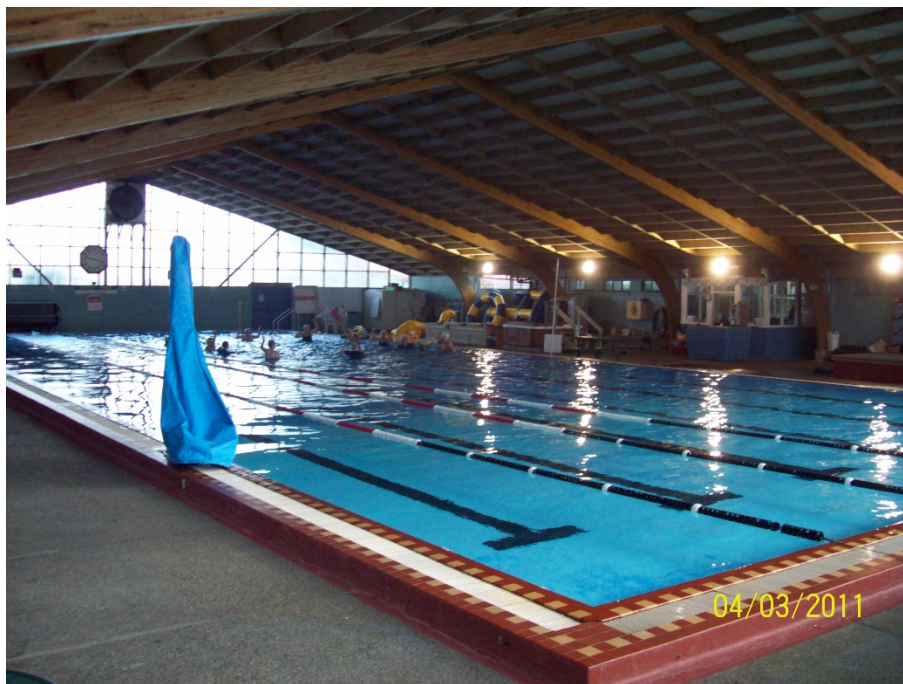
Picture 1: Pool Hall – Insulated Roof & Uninsulated walls
