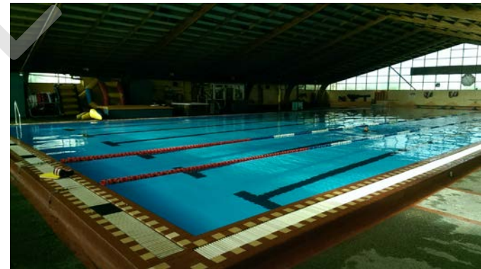
View Looking North East
