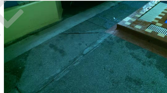
Pool Surrounds - Condition
